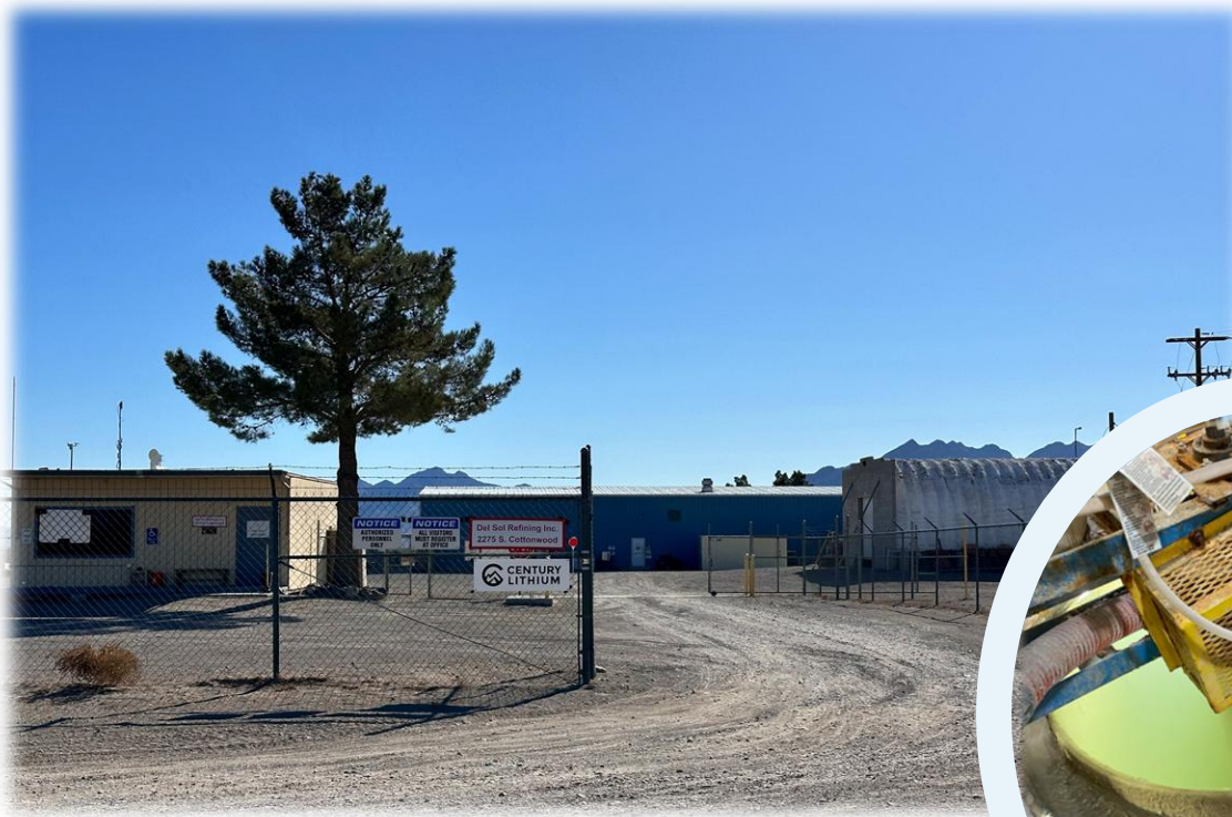
Demonstration Plant Facilities
