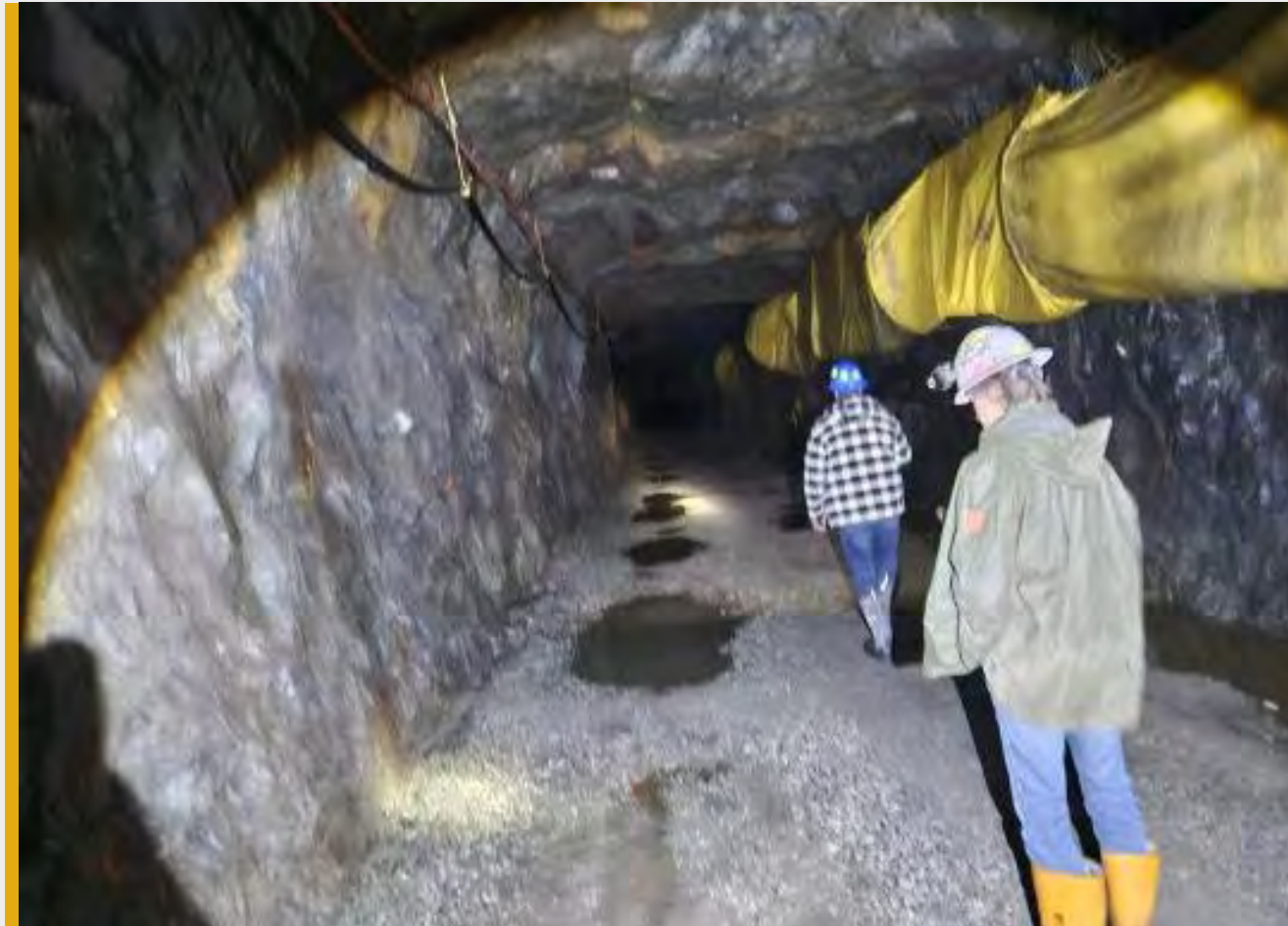
U/G Inspection, 830 level. October 2025
