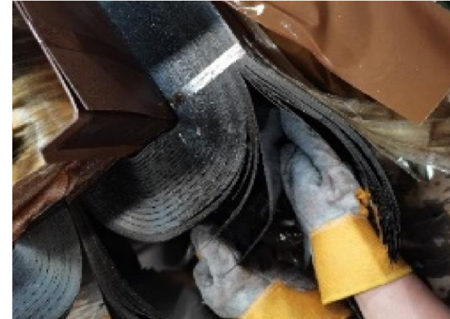
picture: Amorphous transformer core replacement
